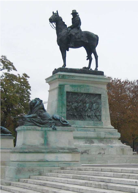
Figure 1: Bronze plaques staining existing Civil War monument base
