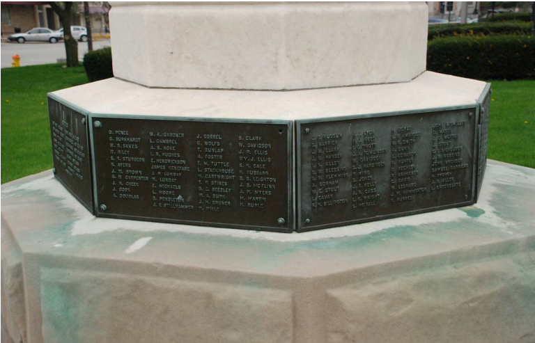
Figure 1: Bronze plaques staining existing Civil War monument base
