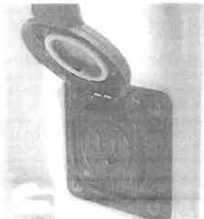
Standard 120-volt power outlet in bed
