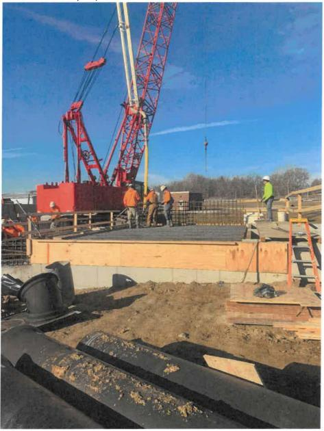
Channels have been poured for the placement of the influent axial flow pumps
