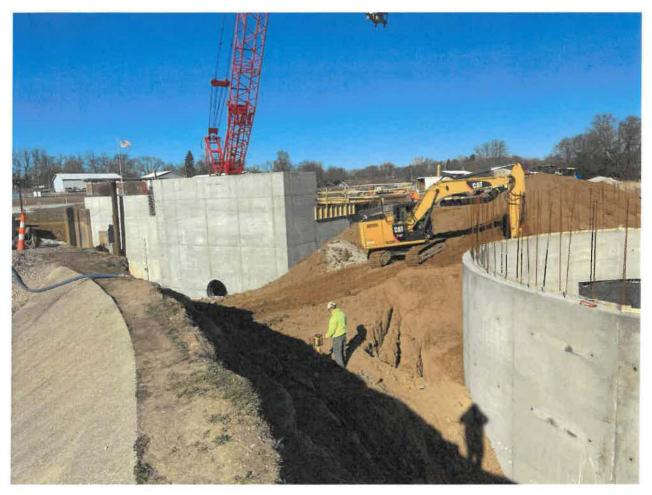
• All of the below grade work on the screen structure has been completed, and now work begins on the area above the pumps
