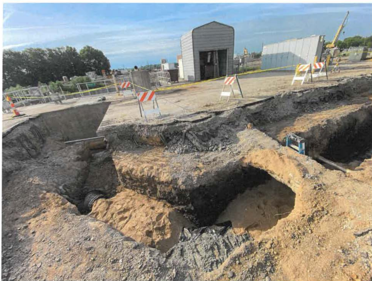
Influent raw water line relocation
