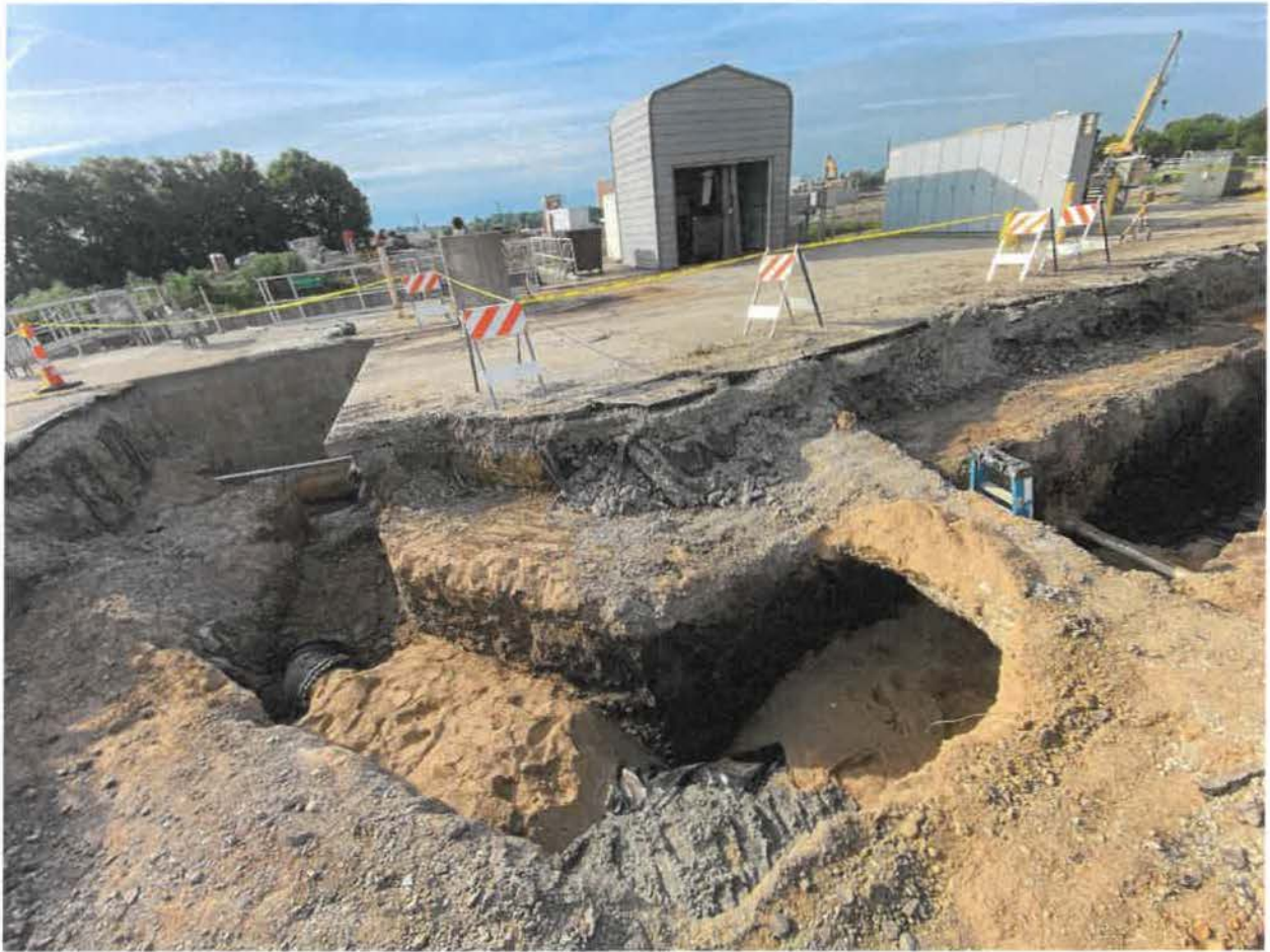
Influent raw water line relocation
