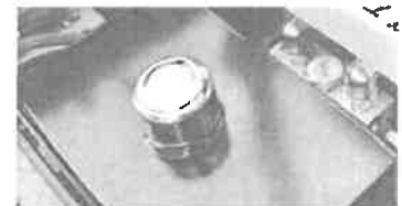
Large Oil Reservoir
